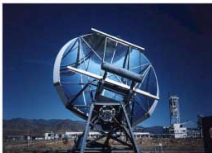
FIGURE 4.6 High concentrating solar collector. Parabolic dish solar collector (PSA, Spain).
