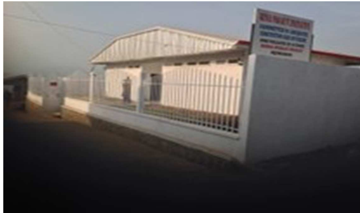
Figure 5. Irina public toilet in the Njinikom open market
