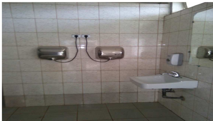
Figure 7. Irina public toilet in the Njinikom open market
