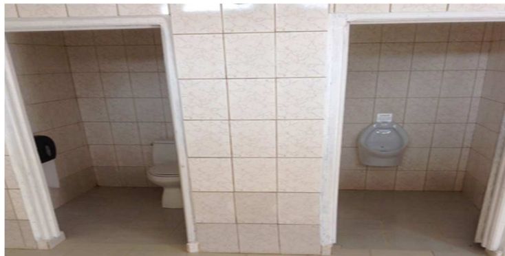
Figure 6. Irina public toilet in the Njinikom open market
