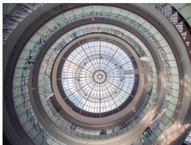
Fig. 1. An example of a large dome-shaped roof where an ellipsoidal reflector antenna for UHF-RFID applications could be integrated.
