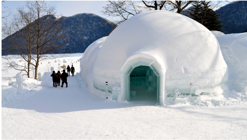
Figure 3: The thermal insulation of an igloo by a layer of snow (photo by David McKelvey on www.flickr.com ).
