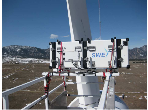
(b) The SWE-LIDAR installed on the CART2.
