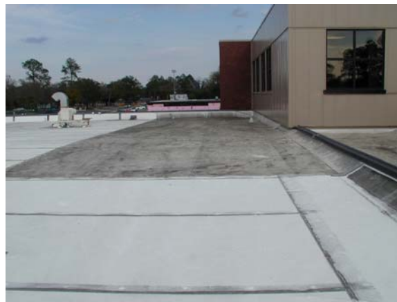
Figure 1. New and Aged Samples of Installed Roofing Membrane.
