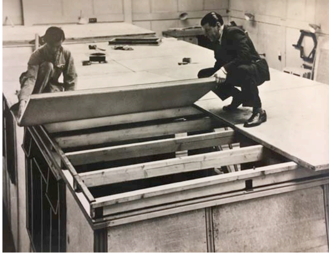
Figure 8.10 Laying the roofing panels. (Airfield Research Group)
