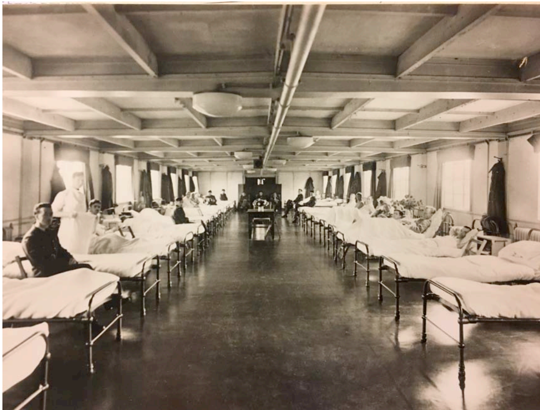
Figure 5.13 The Seco Hut as a hospital. (Photo from Seco: In War and Peace , a brochure held by Airfield Research Group)
