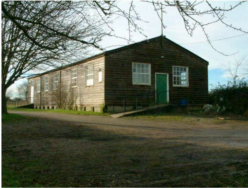
Figure 2.33 Drinkstone Village Hall, a timber Armstrong Type Plan Hut. With thanks to Great War Huts.
