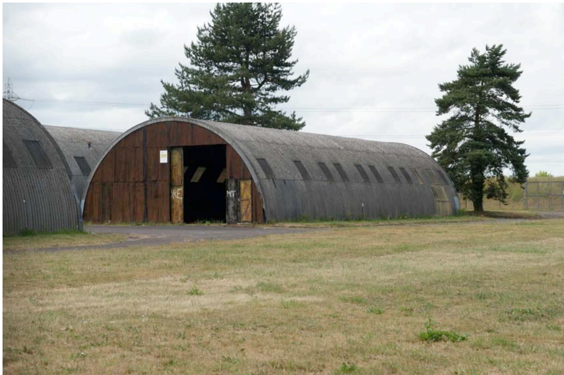
Figure 7.8 A Romney Hut with natural deadlights visible in the corrugated steel sheets. (Airfield Research Group)
