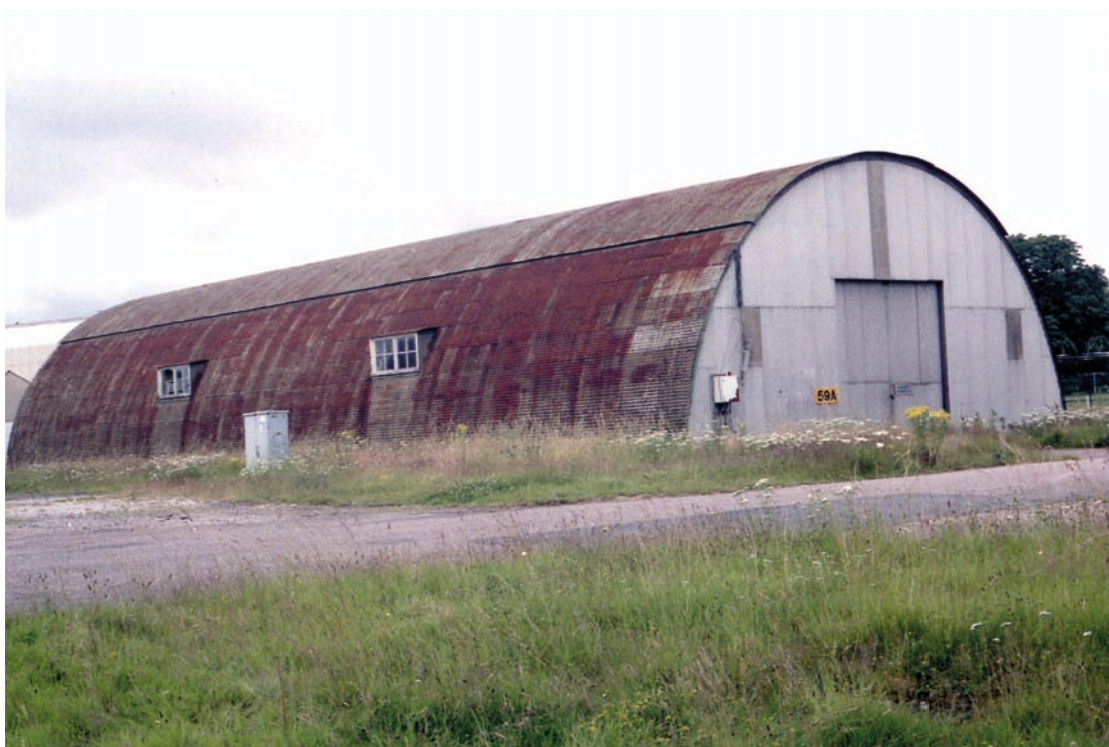
Figure 7.11 A large Quonset hut. (Airfield Research Group)
