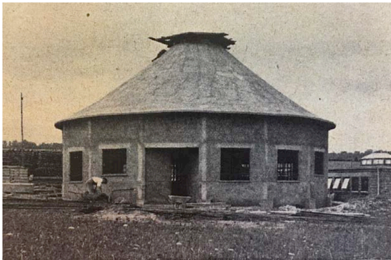
Figure 6.10 The Quetta Hut. The Builder (25 July 1941)
