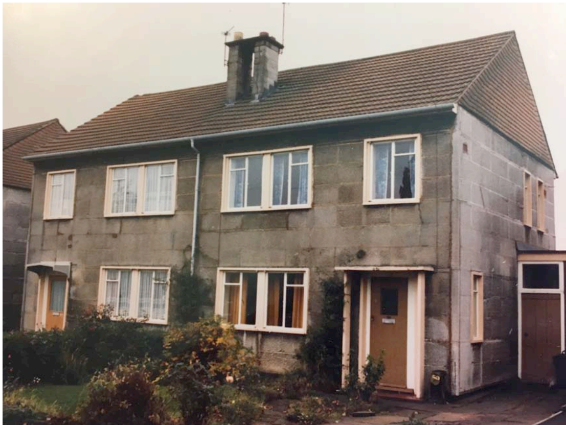
Figure 8.17 The pitched roof Orhit House c. 1990. (Photo by Paul Francis, Airfield Research Group)
