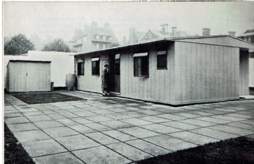
Figure 8.3 The Portal Prefab on display at the Tate Gallery in 1944. (Image courtesy of The Prefab Museum)
