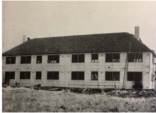
Figure 8.1 The Concrete Clad House erected in less than two weeks at Northolt. Demonstration Houses (1944)
