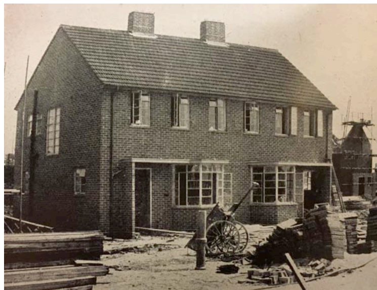
Figure 8.2 The steel-framed brick clad house at Northolt. Demonstration Houses , (1944)
