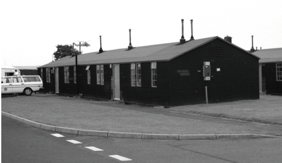
Gerrard & Sons Y Hut at RAF Chivenor. Photo by Paul Francis.
