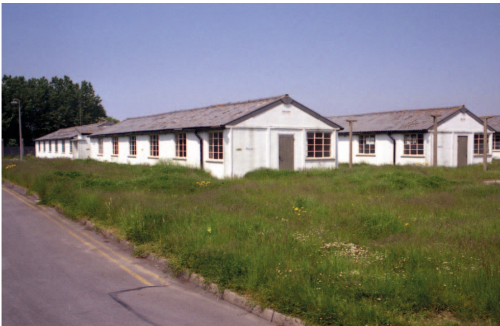
Figure 6.22 Ministry of Works Standard Huts, 18 ft 6 in. span. Photo by Paul Francis, Airfield Research Group.
