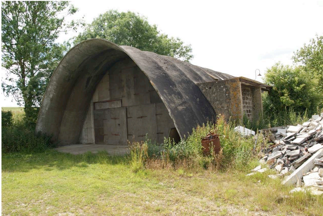
Figure 6.15 A C'tesiphon Hut, Everleigh, Wiltshire before demolition. Photo by Paul Francis (Airfield Research Group).
