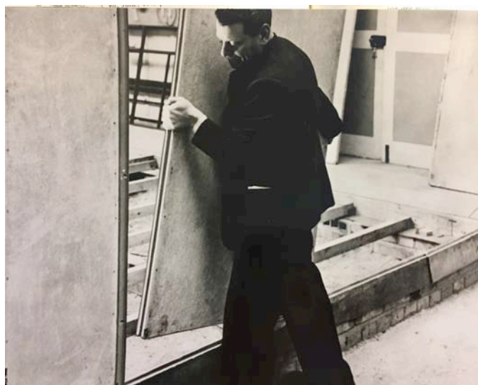
Figure 8.9 A Seco panel is inserted into the frame. (Airfield Research Group)
