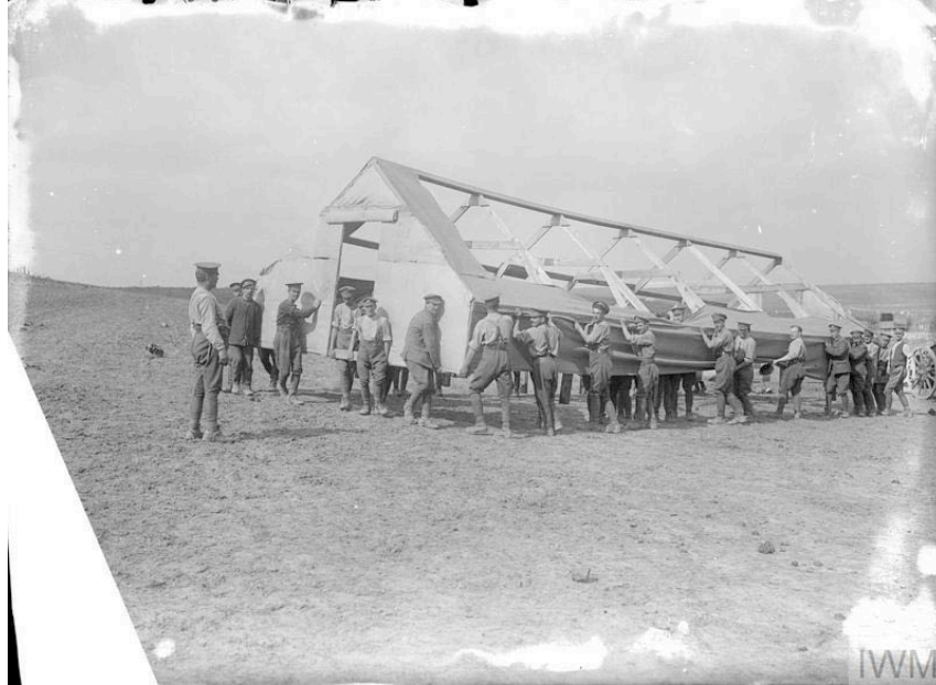
Figure 2.7 Royal Engineers move a hut during the Battle of the Somme, Sept. 1916. It is possible this is an example of one of Armstrong's canvas and timber huts. (© IWM Q1204)
