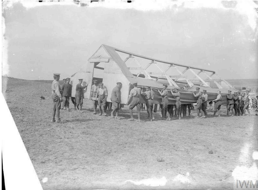
Royal Engineers move a hut during the Battle of the Somme, Sept 1916. IWM (Q 1204) This is possibly an example of an Armstrong Canvas and Timber Hut.
