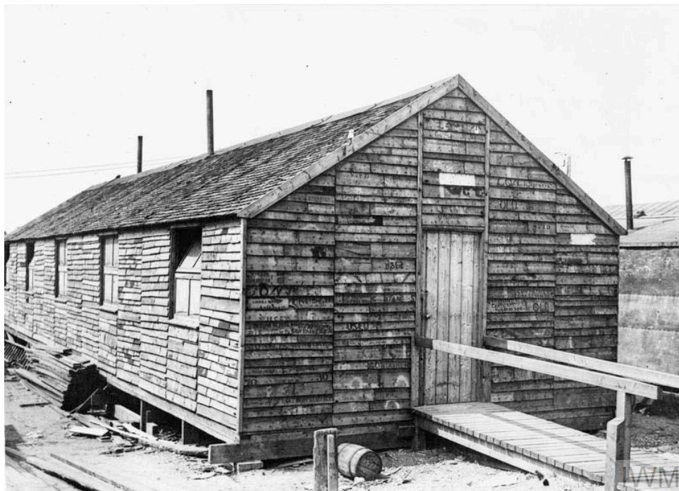
Figure 2.27 The Tarrant Dechets Hut constructed entirely of used packing crates. Built in France by British women hired to work as carpenters by the Tarrant company. (© IWM Q109797)
