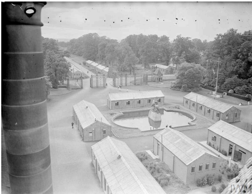
Figure 1 Huts as cadet accommodation at Eaton Hall, Cheshire (c. 1944). This photograph features in Robinson's book Requisitioned , in which the buildings are incorrectly described as being Nissen huts. © IWM A24549
