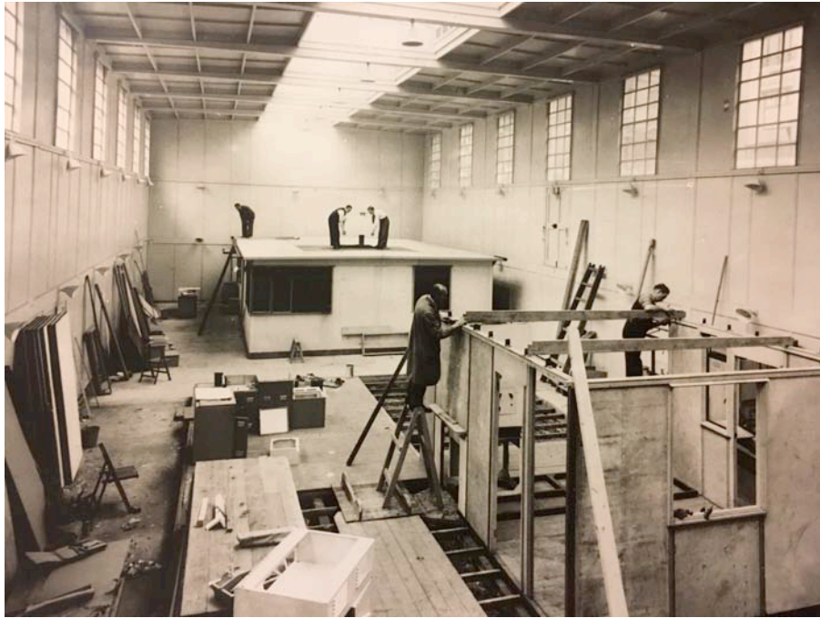
Figure 5.12 Seco Huts being constructed at Uni-Seco Training Centre in London. (Photo from Seco: In War and Peace , a brochure held by Airfield Research Group)
