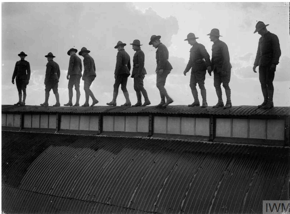
Figure 2.24 Soldiers atop a Nissen Hospital Hut in France. © IWM Q3168
