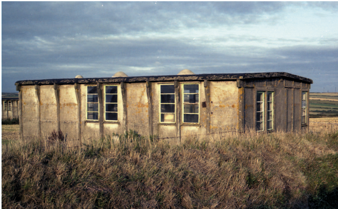
Figure 6.21 A surviving BCF Clear Span Hut. Photo by Paul Francis, (Airfield Research Group).
