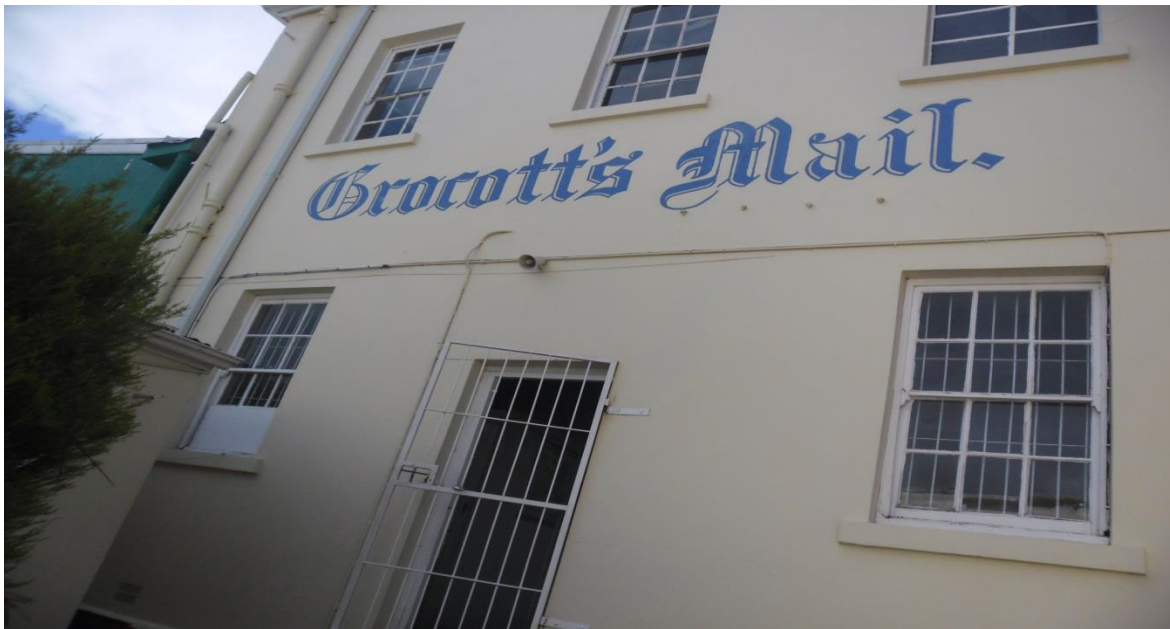
Image 4: The back entrance door of Grocott's Mail Office that houses Radio Grahamstown
