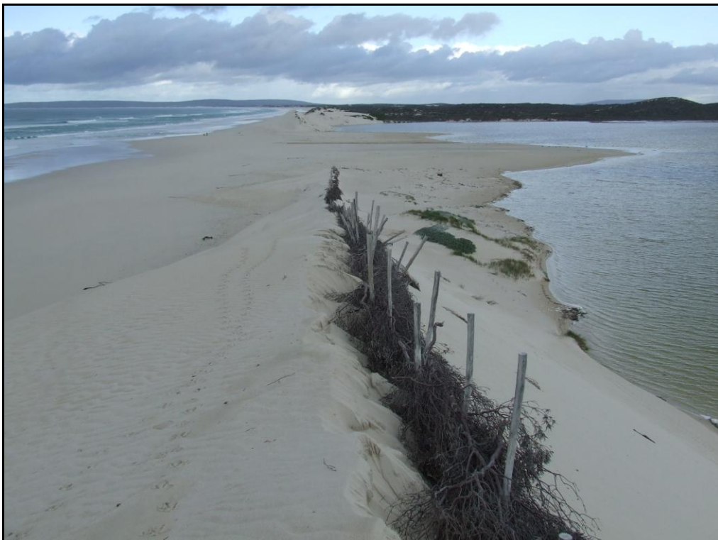
Plate 11 Dune stabilization at the mouth of the Heuningnes Estuary using dried branches of Acacia cyclops .
