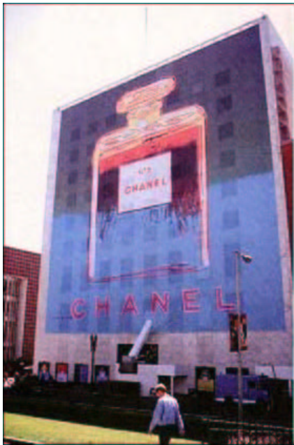
Figure 59. Vinyl mesh panels used to cover a building. (WFDIC, 1998)
