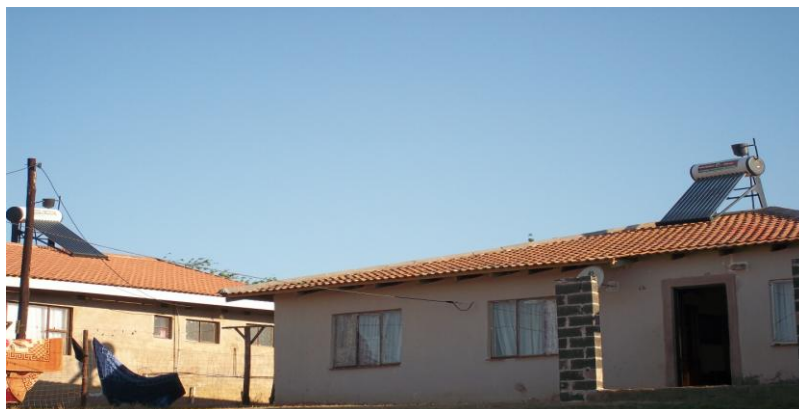
Figure 1: Solar Water Heater Installation in Buffer Strip
