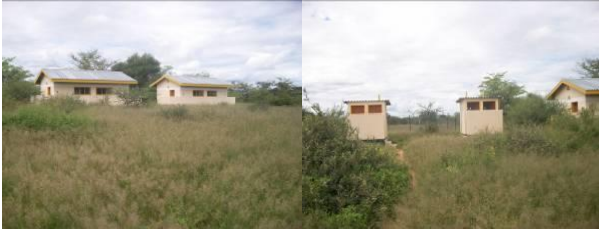
Plate C6.4: Locked water system or flush toilets and pit latrines
