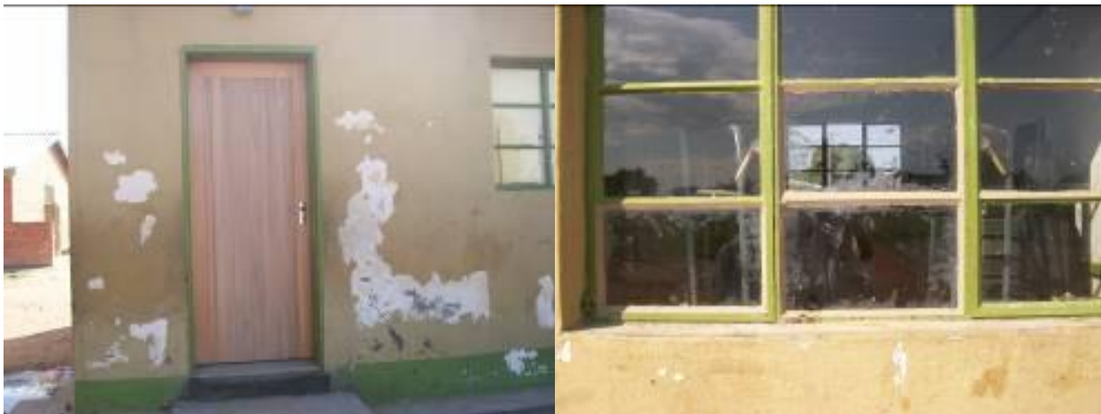
Plate 9.3: New door and fixed window
