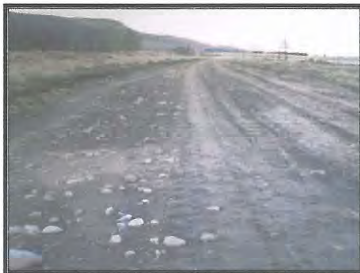
Figure 1.4. An example of a farm road, large boulders and ridges are common.
