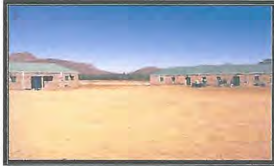
Figure 6.3. The interior (previous page) and exterior (below) of the Khulanathi 26 Centre on NECF property
