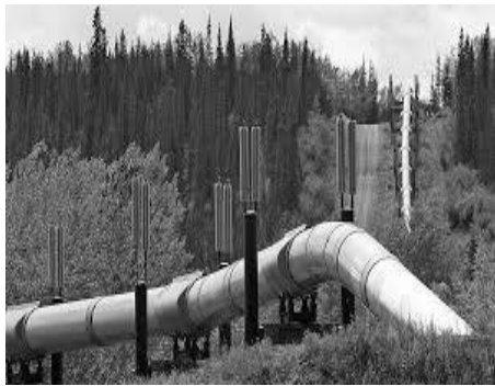
Fig 2: Hydro electric pipelines
