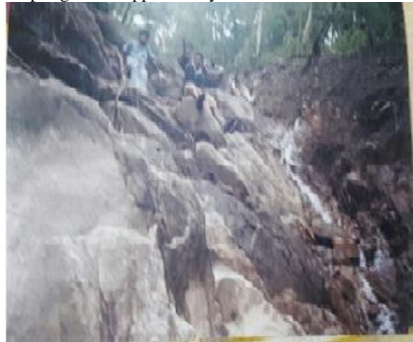
Fig 3b: joints dipping towards the hill slope favouring plane failure (middle portion)
