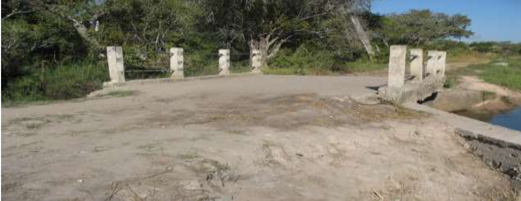
Figure 7: Bridge at Lulimala stream rehabilitated using CRB funds
