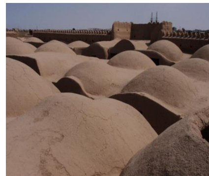
Figure 11. Compacted context of Mehrjard castle
