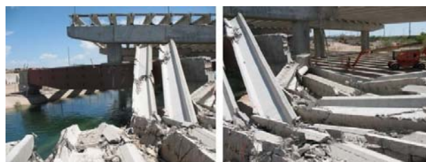
(a) Power Road, Red Mountain Freeway in Mesa, Arizona [1]
