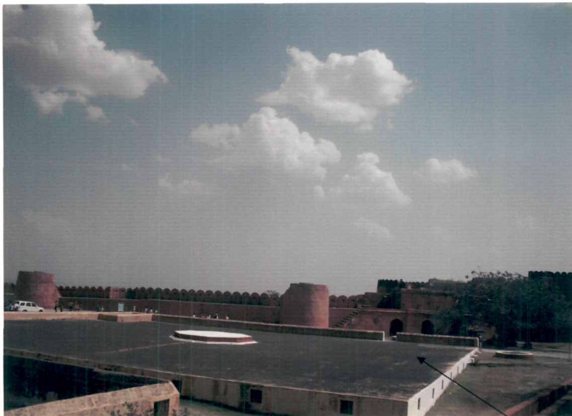
(VIII): Covered Tank of Jaigarh Fort
