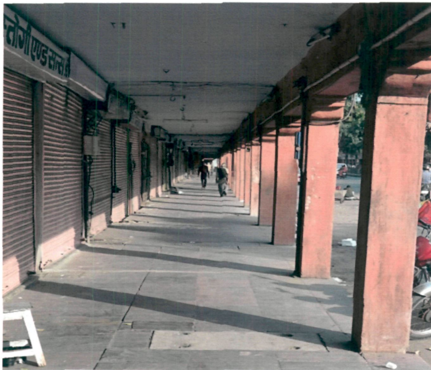
(XIX) Walkway Infront of shop
