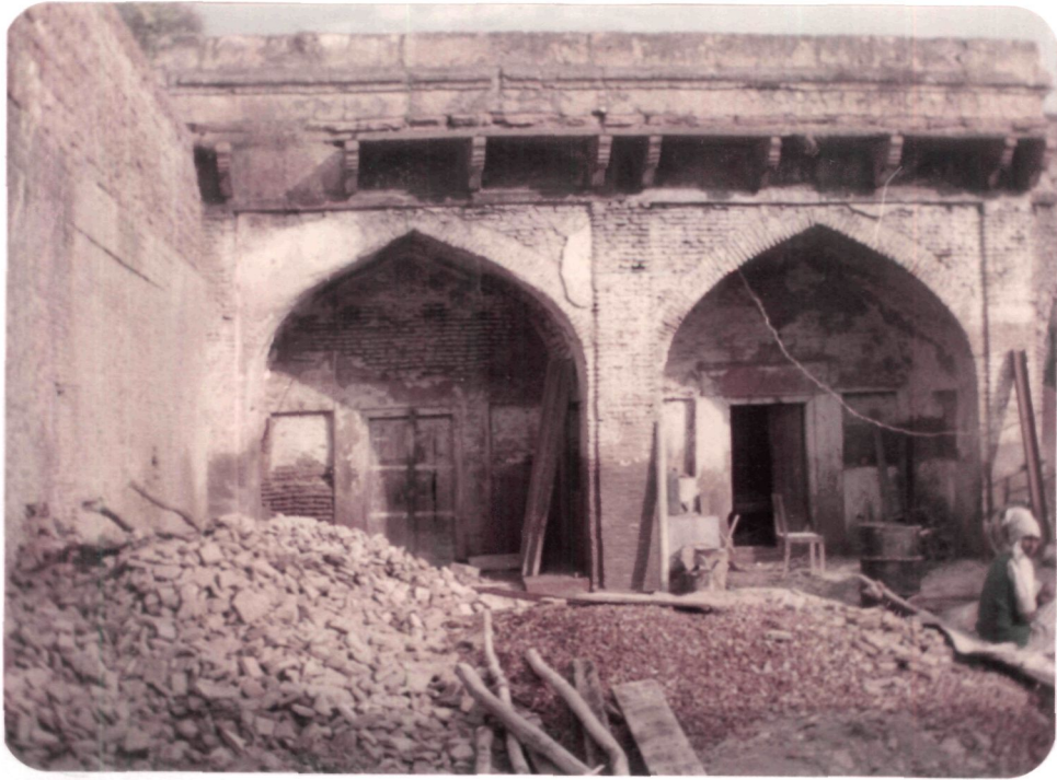
Plate I : A : Cloistered Apartment (Badshahian) at Katra Phulail.
