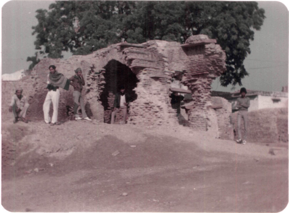
Plate II : A ; Pukki Sarai : view of a ruined apartment.
