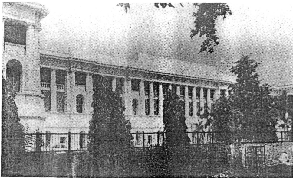
Fig. 59. Western Court and Eastern Court
