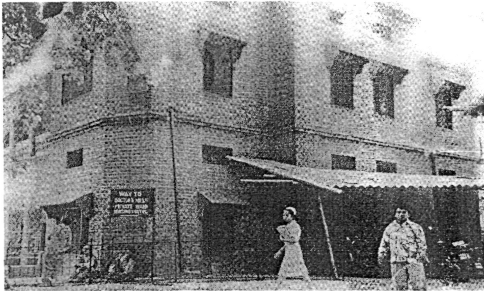
Fig. 14. HOSPITAL VICTORIA ZANANA
