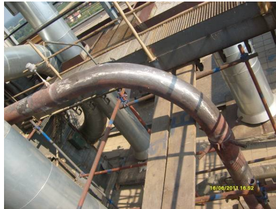
Figure 1: Part of the steam line during NDT.
