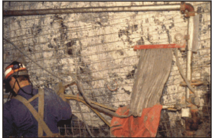
Figure 5.—Underground storage of fire water hose in a rack.
