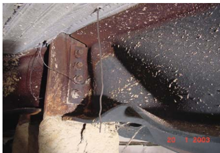
Fig. 19. Beam web in shear.
