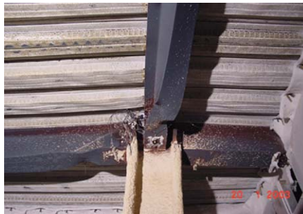
Fig. 18. Local buckling of beam lower flange.
