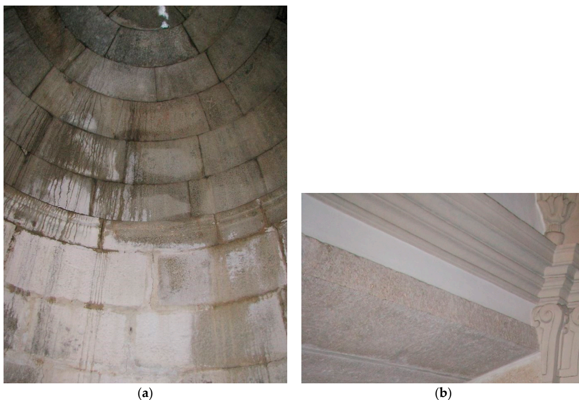
Figure 1. Images illustrative of the indoor space typology: (a) type A spaces, where granite is the dominant material in all the space elements (floor, walls, ceiling); (b) type C spaces, where there are granite applications but other materials are as abundant as or more abundant than granite.
