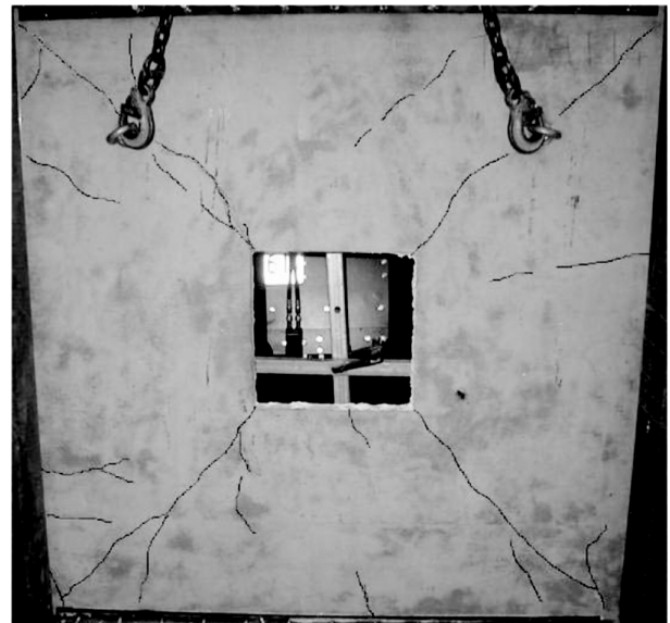
Figure 11. Crack pattern on tension face of T45W1C1.4
