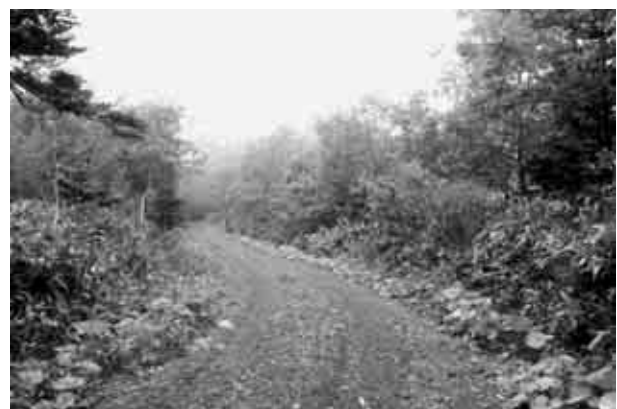
Figure 1 Well maintained main forest road (Maeyama, constructed in 1968. Base rock is welded tuff.)
