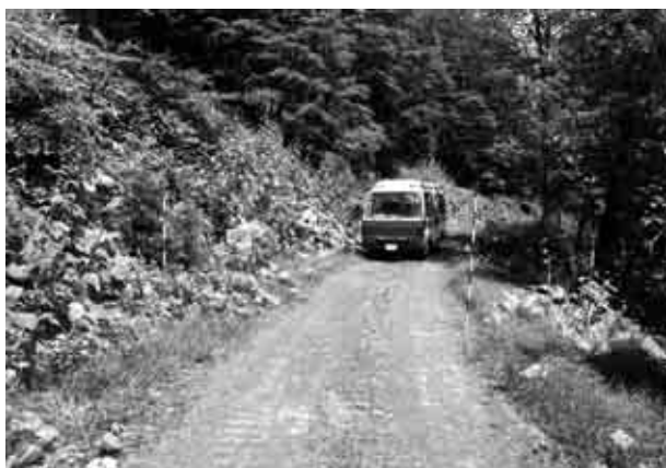
Figure 2 Well maintained main forest road (Higashiyama-honryu, constructed in 1967. Base rock is welded tuff, metamorphic green rock andecite. Pavement is shale stone.)
