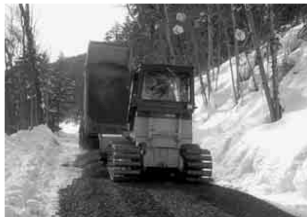
Figure 3 Maintenance (Gravels are supplied for the surface of pavement. The average volume of gravels is about 0.49 \text{ m}^3/\text{m} .)
