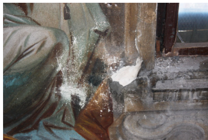
Image 98: Efflorescence, superficial erosion and lacuna
