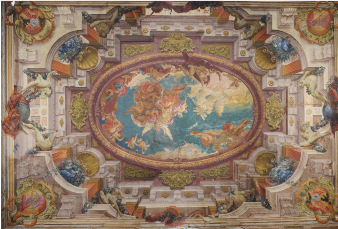
Image 38: False ceiling of the ballroom
