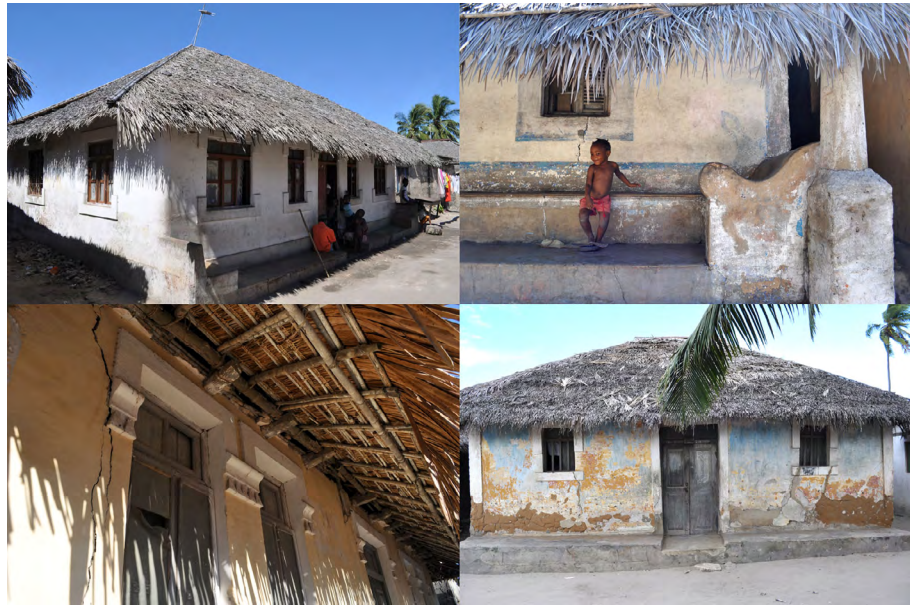
Illustration 2: Macuti houses in Ilha de Moçambique, some with cement walls and macarasse leaves instead of macuti roof cover
