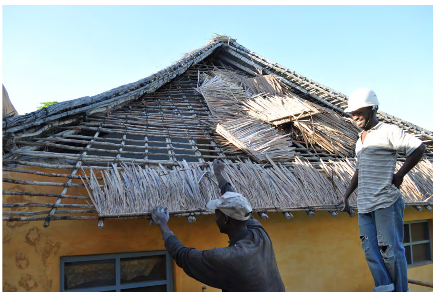
Illustration 7: Improved macuti roof construction using double tiles
