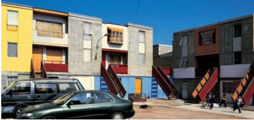
Fig. 13: Distributed design: Top: The housing scheme at the time of delivery (the architect's completion). Bottom: Same view one year later after additions by the occupants. Alejandro Aravenas: Elemental - Quinta Monroy. Photo: Christobal Palma
