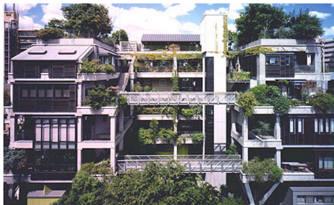
Fig. 14 Top: Le Corbusier's 'plan libre' in the Maison Domino proposal, 1913. Radical freedom for users, but not built. Bottom: Utida 1993, Next 21, boliger i Osaka. Built, but not transformed. Photo: http://www.arch.hku.hk/~cmhui/japan/next21/next21-index.html#4 .
