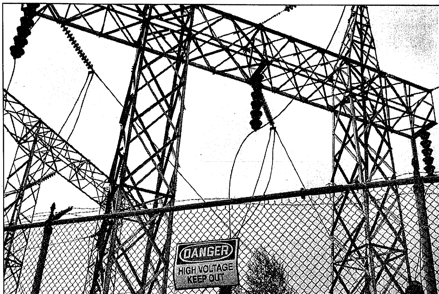
THE POWER lines running into the Kitimat aluminum smelter carry electricity generated at Kemano using the water of the Nechako watershed. Some say the agreement that gave Alcan the use of that public resource is being perverted. MATTHEW PETERSON PHOTO
