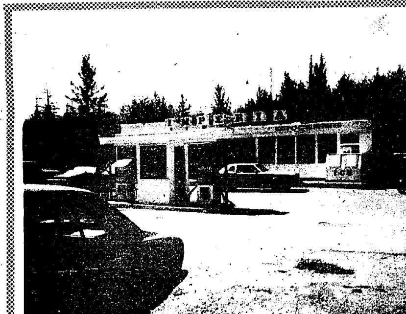
Well located service station corner grocery complex. Ideally set up for family operation.
