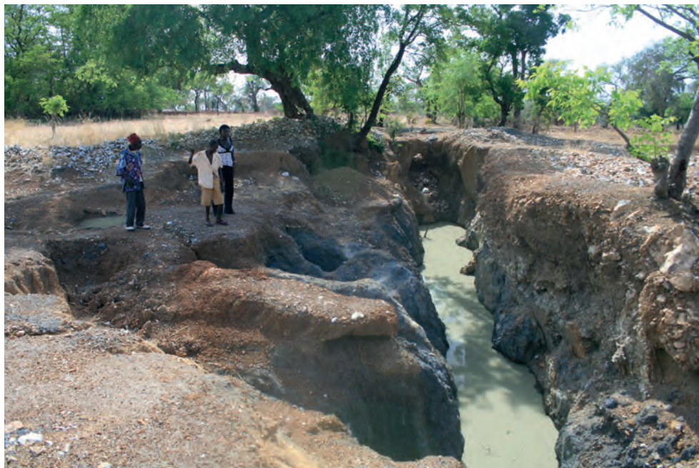
Figure 6.3: The Tingandem and his assistant inspect the damage of illegal mining activities, Tancharra, Ghana. Source: Bas Verschuuren.
