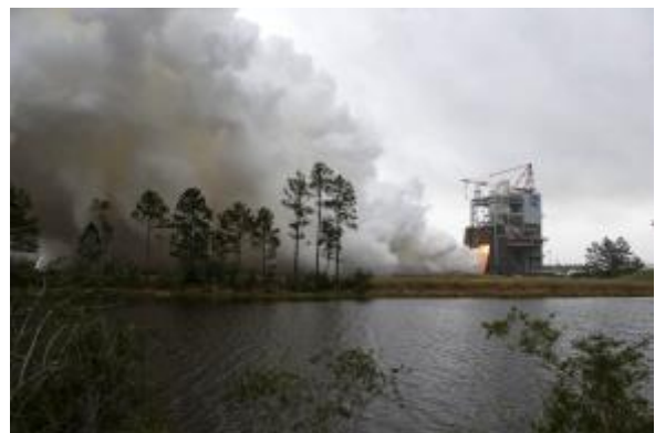
Figure 3. RS-25 testing at Stennis Space Center.
