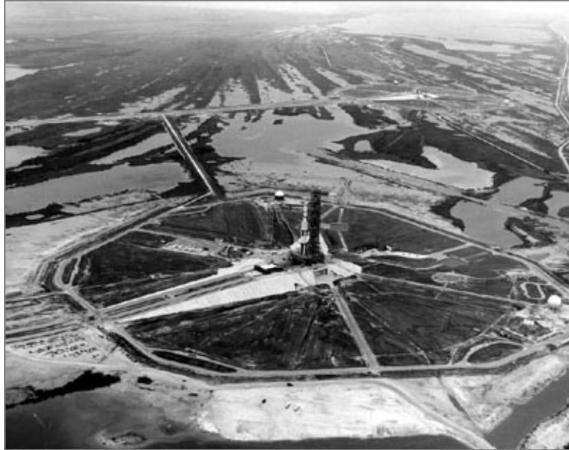
Figure 5. Launch Pad 39. Depicts the propellant storage spheres, the Pad apron, perimeter road, and the Apollo-Saturn V-Mobile Launcher stack.
