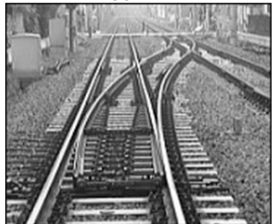
Fig. 1. Railway tracks to be moved by a turnout system
