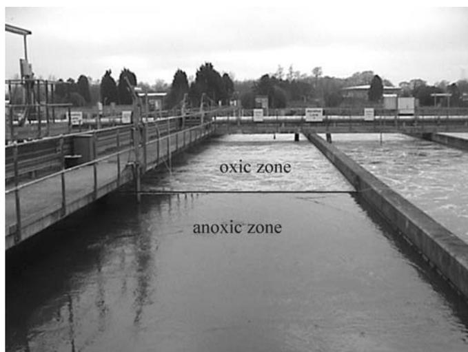
**Figure 2: Activated sludge aeration lane at Finham**
