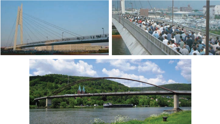
Figure 2.5: Toda Park Bridge in Toda City, Japan (top) (Pictures from Nakamura and Kawasaki (2006, 2009)) and a steel arch footbridge across Main at Erlach, Germany (bottom).
