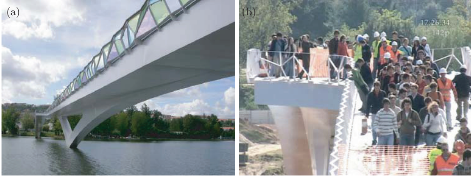
Figure 20: Coimbra Footbridge (a) and pedestrian crowd tests (b) (Pictures from [108])
