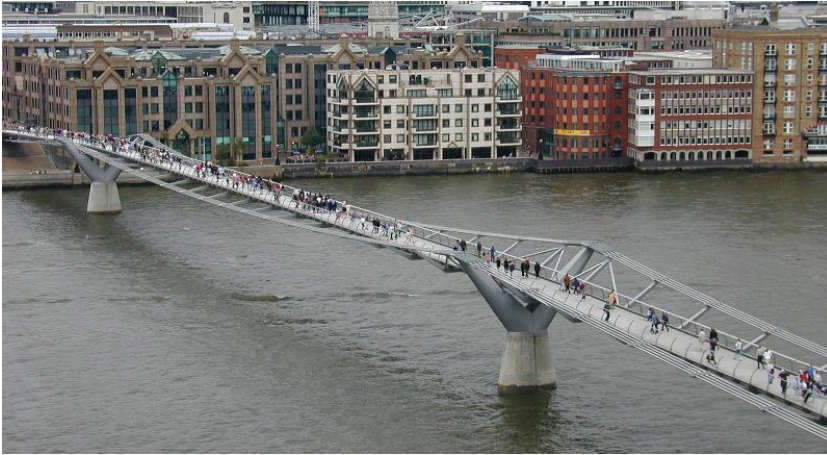
Figure 1.1: The London Millennium Footbridge (Picture from http://www.cambridge2000.com/gallery ).
