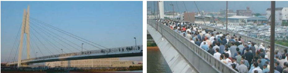
Figure 1: Toda Park Bridge in Toda City, Japan (T-Bridge). (Figures from [40] (left) and [41] (right))
