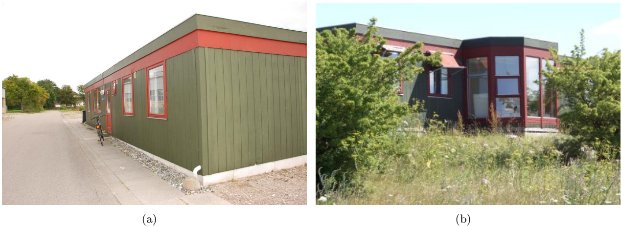
Figure 3: (a) the north facade and (b) is the south facade of the building.
