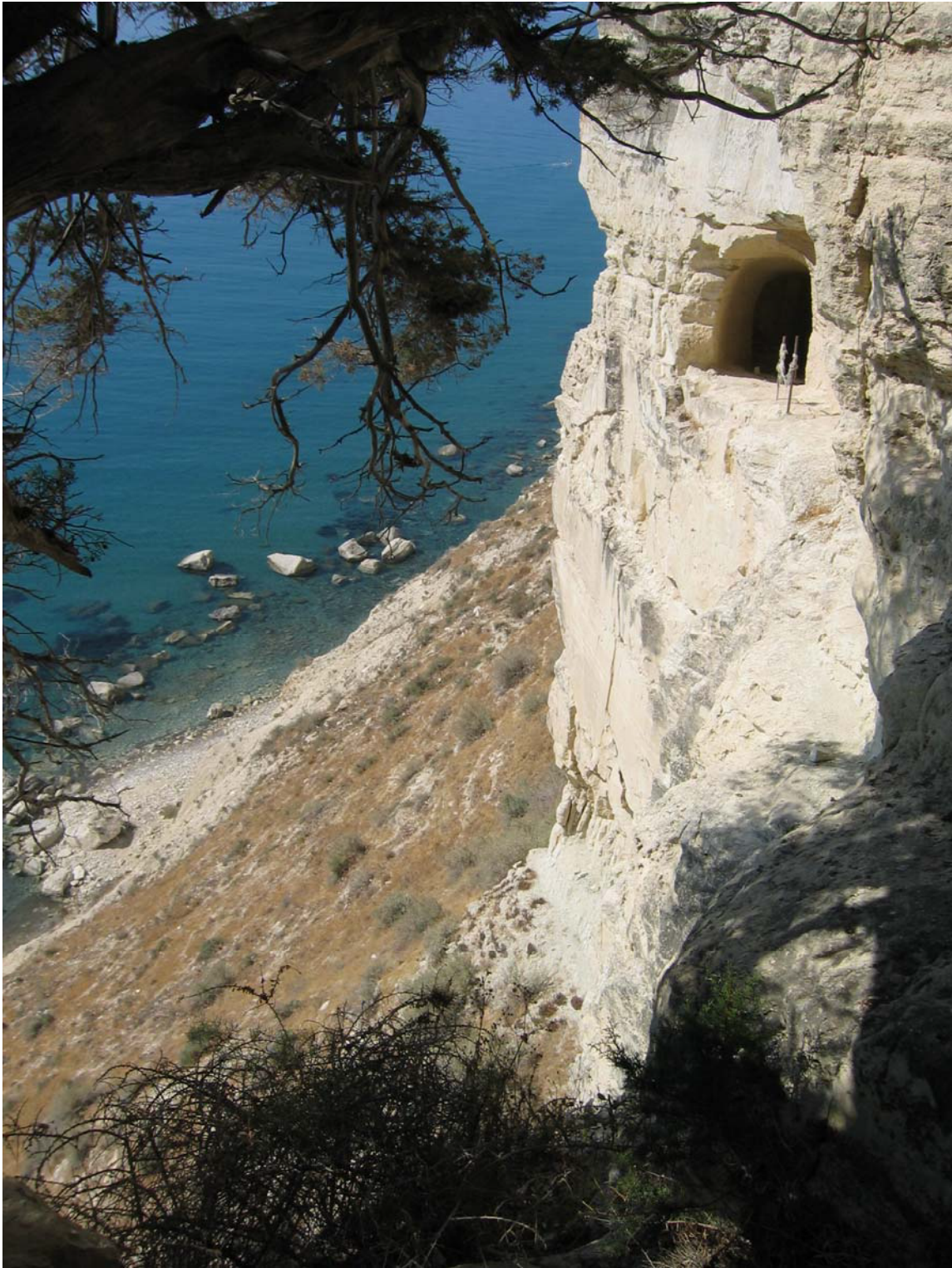
Fig. 2.4 Tunnel at Number Three Bay looking southwest.
