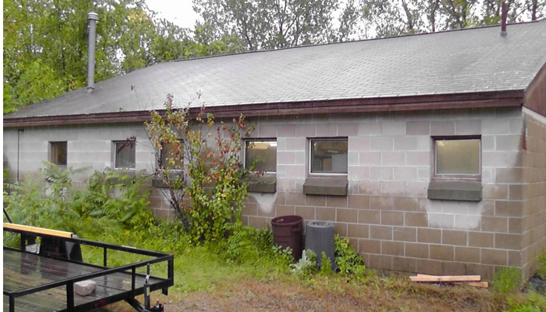
Figure 14: Exterior of Existing Structure
