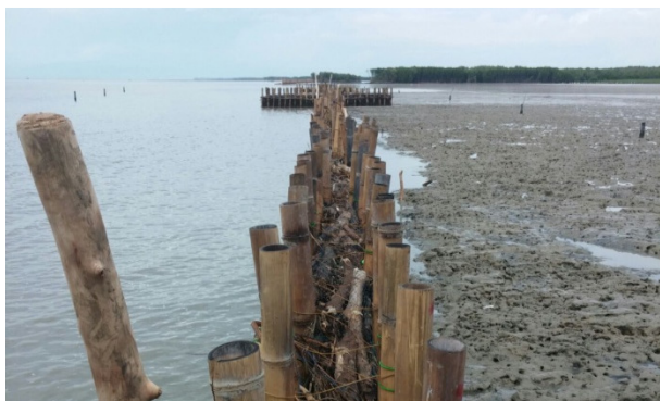
Figure 8 Permeable structure a few months after construction. At the landward side (to the right) sediment has settled above low water.
