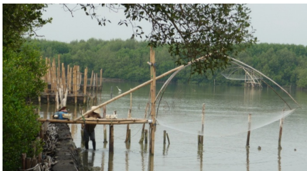
Figure 10 Villagers have constructed their own fishing platform in the shallow waters near the permeable structures to have an alternative livelihood.
