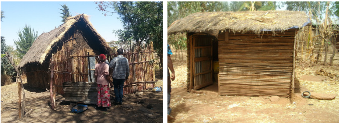
Figure 2: Examples of village poultry houses constructed from locally available materials.
