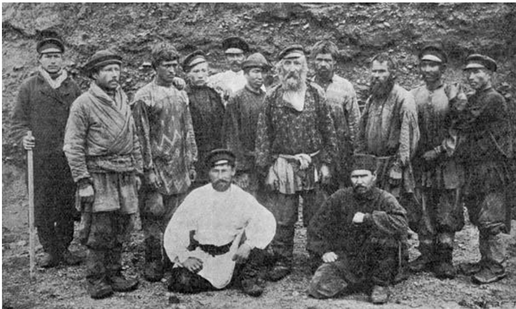
Figure 2 A group of Trans-Siberian workmen at the construction of the Trans-Siberian railway (1898) Available at: http://www.transsib.ru/Photo/Old/old-237.jpg
