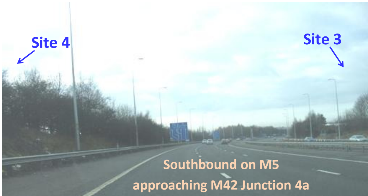
Fig. S1d. M5 motorway crossing Battledfield Brook between Sites 3 and 4.
