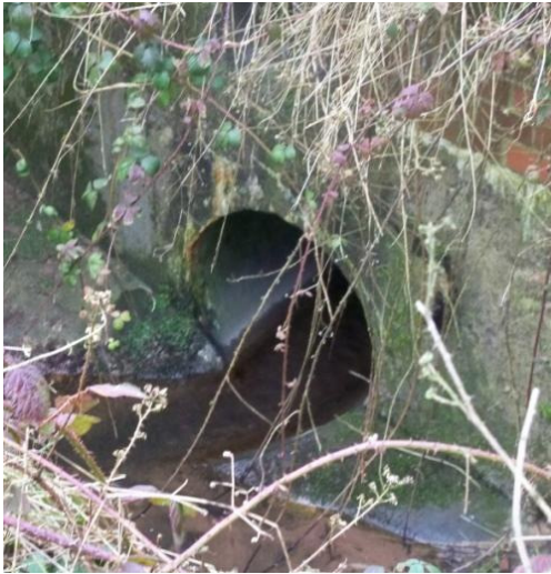
Fig. S1g. M5 motorway runoff pipe discharges to the Battlefield Brook between Site 1 and Site 2 (left) and Sites 3 and 4 (right).
