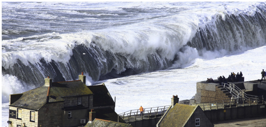
Fig. 1. Wave breaking directly on Chesil beach during storm on 5 February 2014; the flow just landward of the large collapsing breaker is best described as backwash. (photo by Richard Broome, reproduced with permission).
