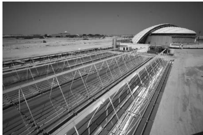
Fig. 7 Use results of Leaner Fresnel type collector (Qatar)
