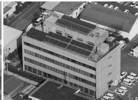
Fig. 9 Use example of triple effect hybrid solar cooling system (Japan)
