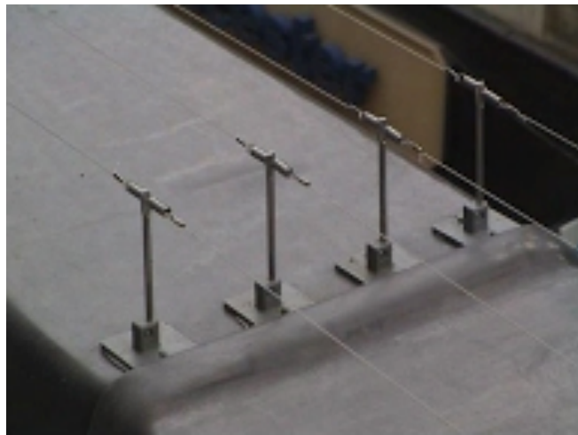
Figure 13: Example of a bird trip wire system installed on a building ledge (Absolute Pest Control Ltd., n.d.)
