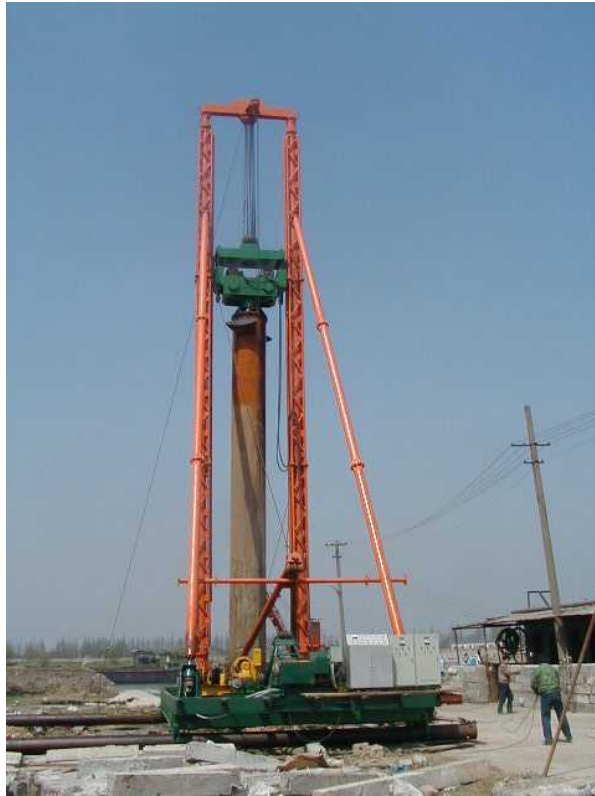
Figure 3 Picture of PCC piling machine
