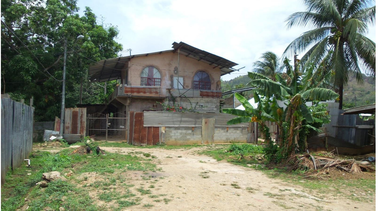
Figure 3. A house at the end of a dirt road in Belleton
